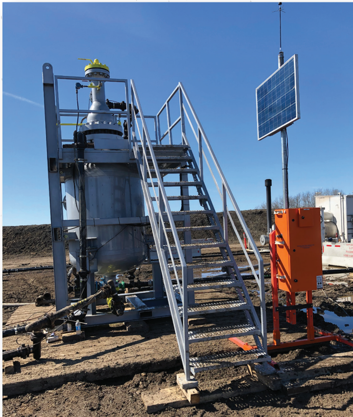
MegaPOL install with Sand Sentry
